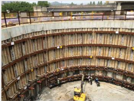
Instrumentation and monitoring for deep excavation
