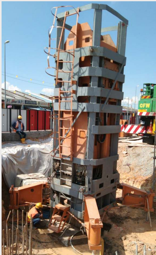
HSDLT with 60tonnes of hammer
