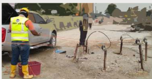
A typical ultrasonic cross-hole testing.
