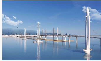
TNB monopole transmission tower Penang
