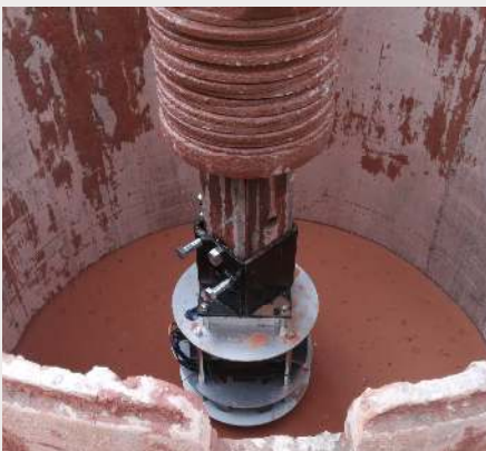
The SHAPE is lowered down into the bored hole with Kelly Bar
