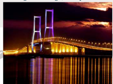
Suramadu Bridge, Indonesia
