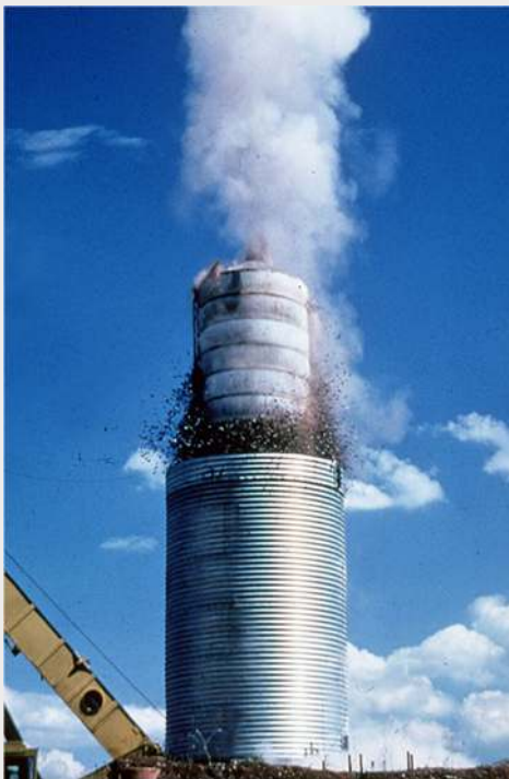
Launching of Statnamic Test
