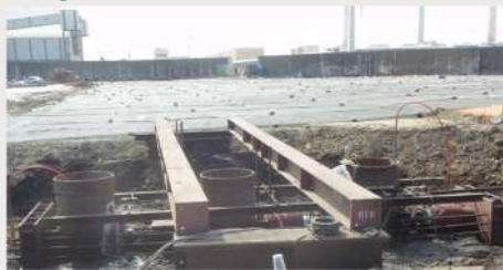
Lateral pile load test monitoring
