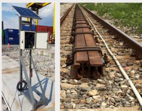
Shape Accel Array (SAA) system
