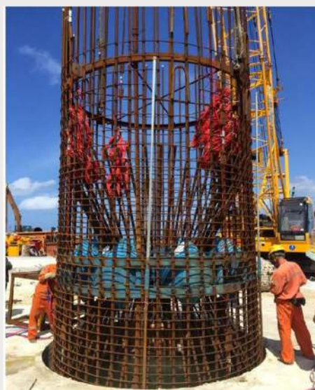
Installation of bidirectional cell inside the reinforcement cage
