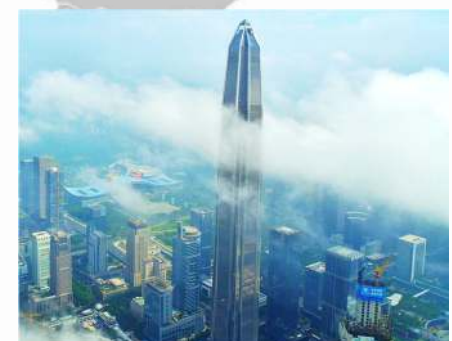
Shenzhen - PingAn International Finance Centre, China
