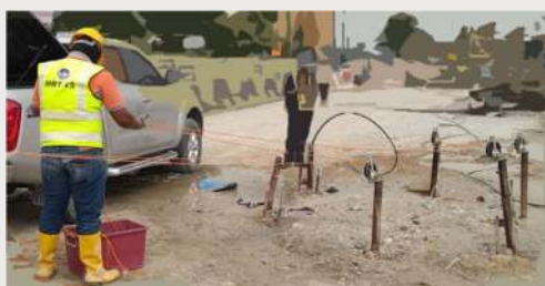
A typical ultrasonic cross-hole testing.
