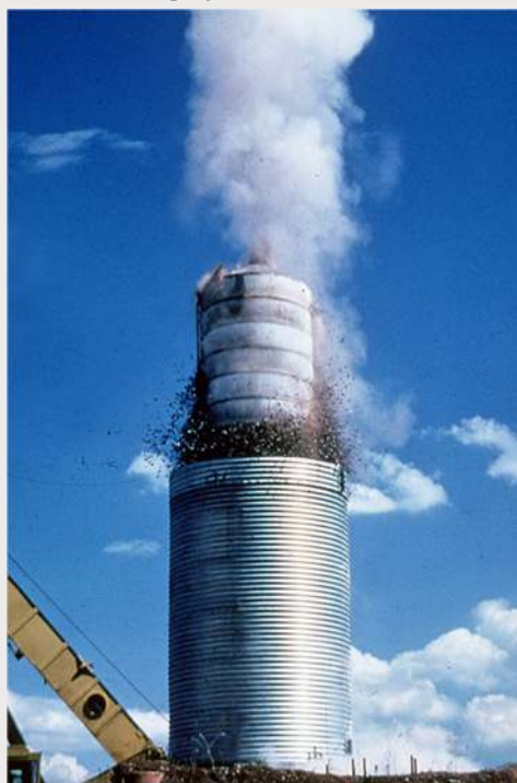
Launching of Statnamic Test
