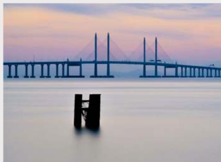
Penang 2nd Bridge, Malaysia
