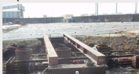
Lateral pile load test monitoring
