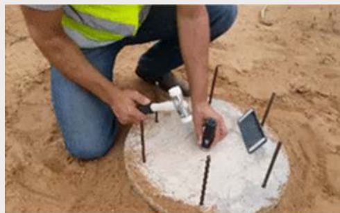
Low strain dynamic pile test
