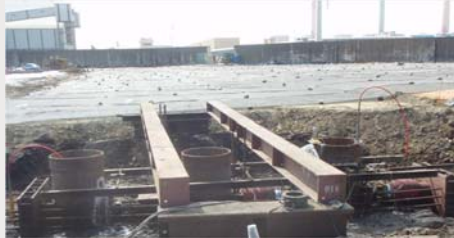
Lateral pile load test monitoring
