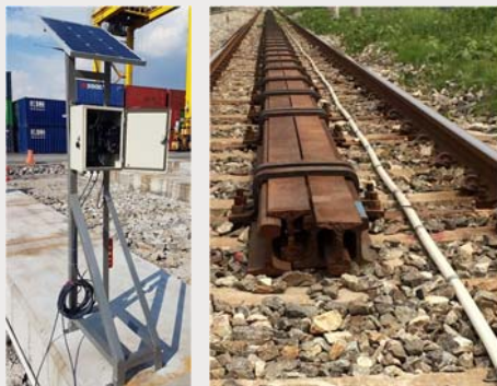
Shape Accel Array (SAA) system
