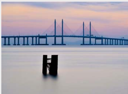
Penang 2nd Bridge, Malaysia
