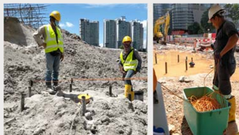
A typical ultrasonic cross-hole testing.
