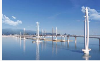
TNB monopole transmission tower Penang
