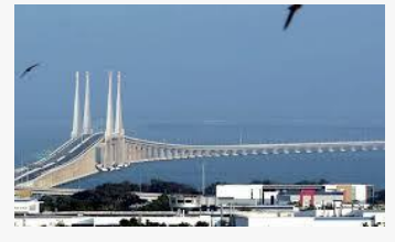
Penang 2 nd Bridge Project
